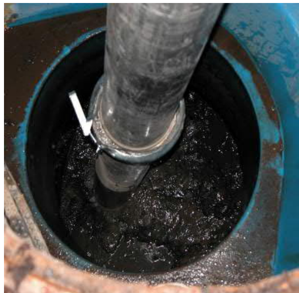
Figure 4: Ensure no blockage for vacuum line
