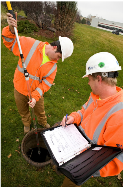
Figure 1: Inspect at grade
