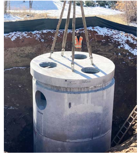
Step 3: Place top slab with access holes.
