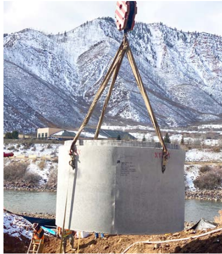
Step 2: Lift and place middle riser.
