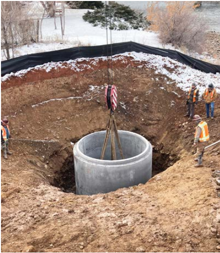
Step 1: Install the base section.
