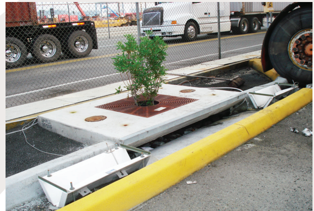
Filterra™ monitoring unit at a port.
